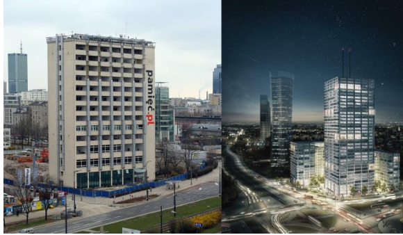
Fig. 5. Photo of IPN's Building for a while before demolition and visualization of Generation Park [Source: [17,19]
