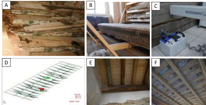
Fig. 2. Recovery of timber structural beams
