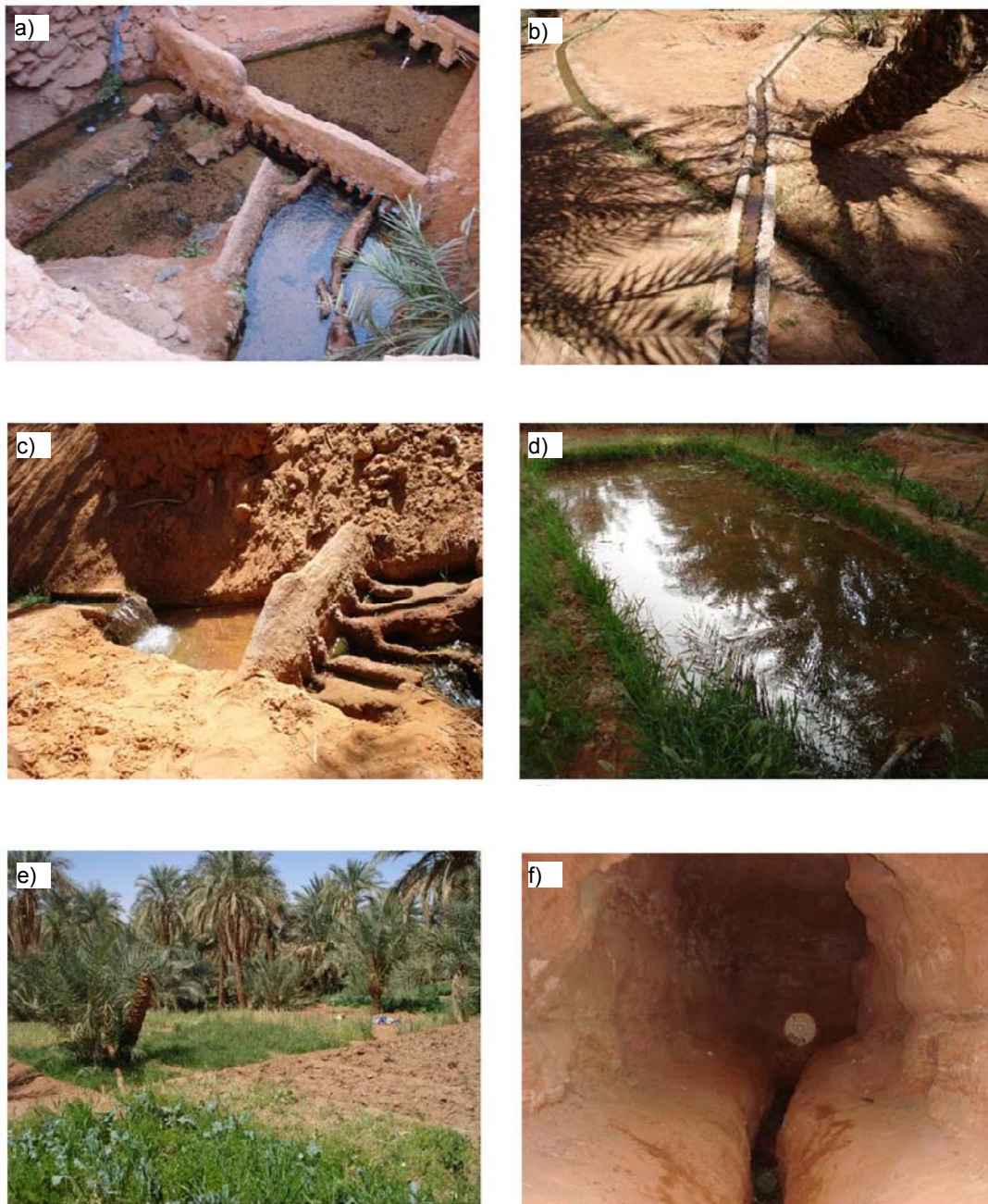
Photo 1. The different parts of a foggaras: a) The main kasria of El Meghaier foggara in the oasis of Timimoun; b) Seguias of El Meghaier foggara to bring water until Madjen in the oasis of Timimoun; c) Secondary kasria of La Salma foggara in the oasis of Timimoun; d) Madjen (tank) of La Salma foggara in the oasis of Timimoun; e) Guemoun (garden) in the oasis of Timimoun; f) A section of the non-active part of the gallery of the foggara of La Salma (phot. B. Remini)
