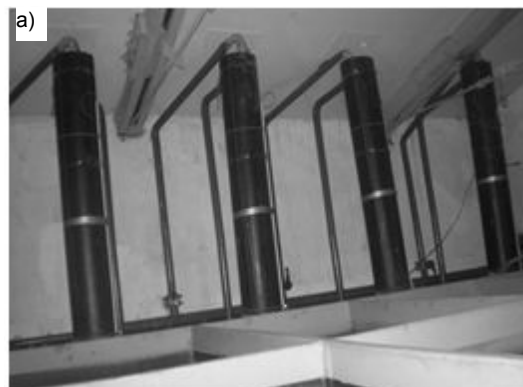
Phot. 1. Contact polystyrene foam filters of Teteryv River water treatment: a) top view; b) flushing valve with pneumatic actuator (photo: S. Martynov)
