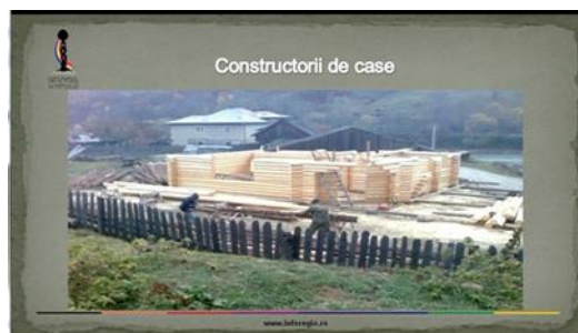
Plate 4 ( SLH , wooden house being built)
