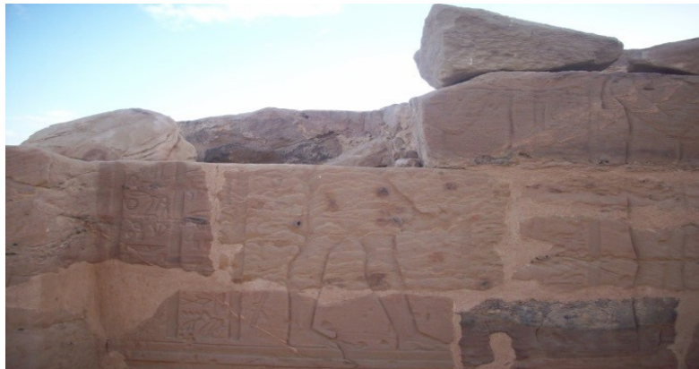
Fig.10. Original Text stone insets that have been lost leading to cavities, with the original stone still in the vicinity
