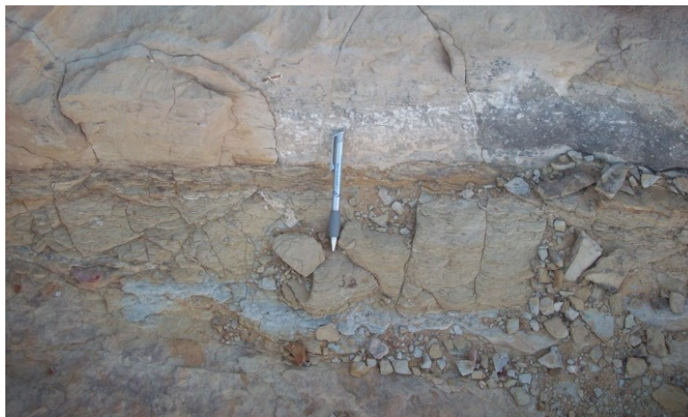
Fig. 14. Detachment of small, flat, thin pieces of the outer layers (Flaking) of El-Nadora Temple stones
