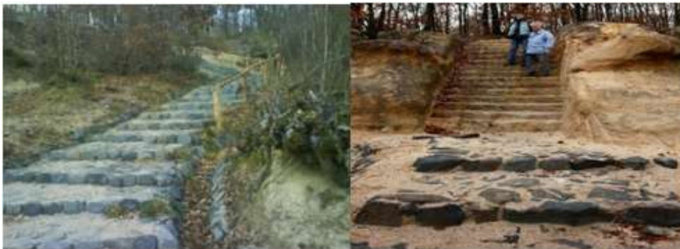
Fig. 30. Realization of successive stairs, photo Aurica Grec, 2015
