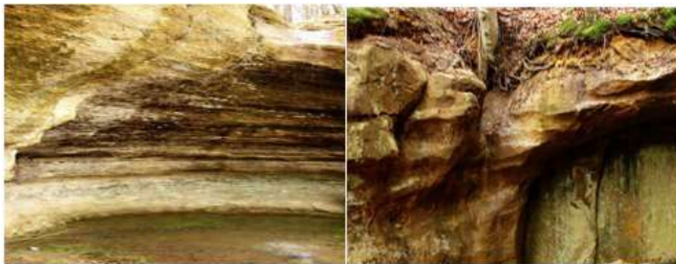
Fig. 28. Figure 2. Mining gallery, photo Aurica Grec, 2015
