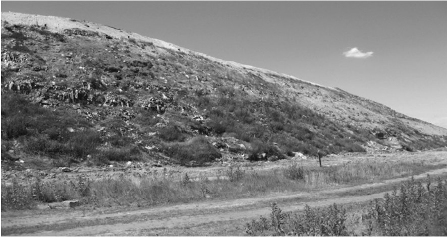
FIGURE 8. The eastern slope of the landfill before reinforcement works
