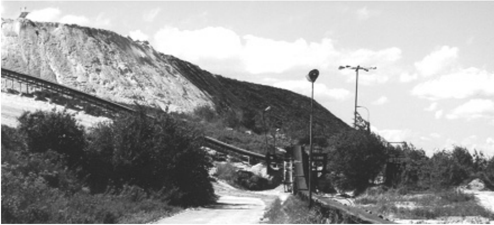
FIGURE 4. Hydroseeding method applied on the phosphogypsum waste dump in Gdańsk Phosphorus Fertilizers Factory – North slope
