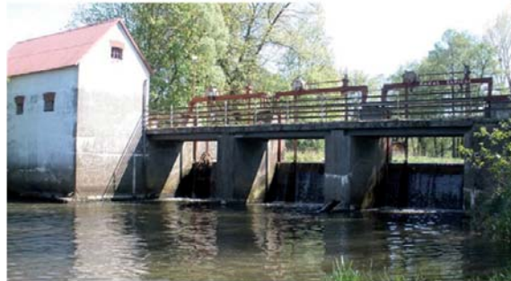
Small hydropower plant in Kamion village (km 37.8).
