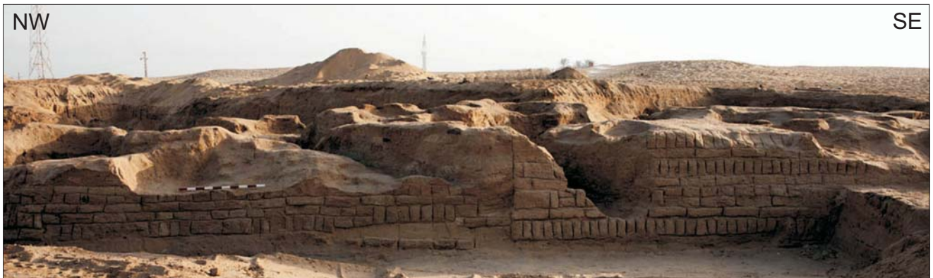
Fig. 2. Outer face of “Wall 1”. Photo by S. Rzepka.
