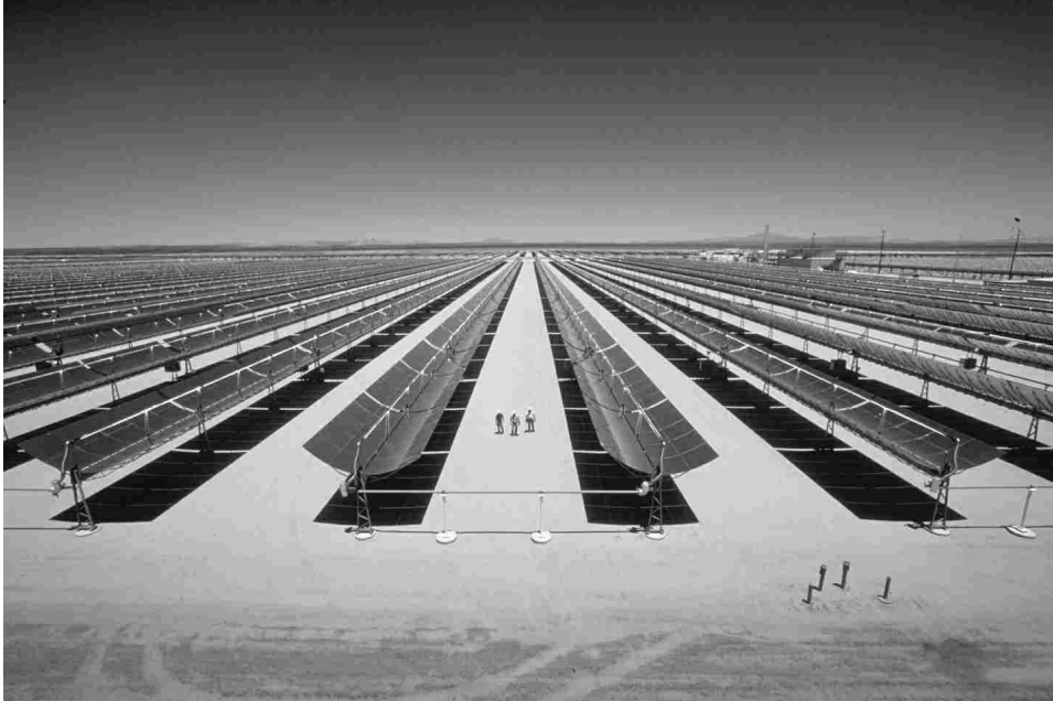
Fig. 1. Concentrating solar power plant with parabolic mirrors in California.
